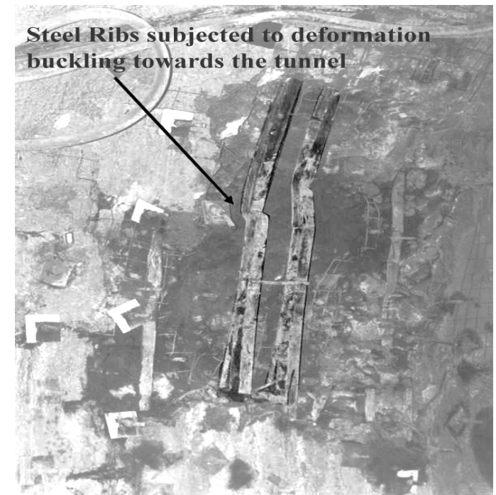
Figure 4. Photograph for tunnel profile at the fault gauge clay where deformations were excessive (Elmalık Left Tube, HEB-100, 20.4kg).
