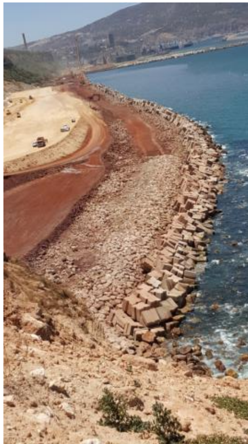
Figure 19: End of the revetment in the construction site (under construction)
