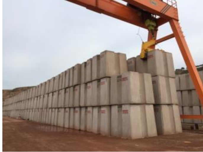
Figure 18: Antifer stocking site in Oran highway construction site
